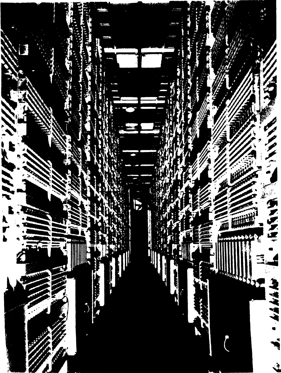
FIG. 14. AN AISLE OF A CENTRAL OFFICE IN A DIAL SWITCHING AREA SHOWING COMPLEXITY OF MODERN TELEPHONY.
